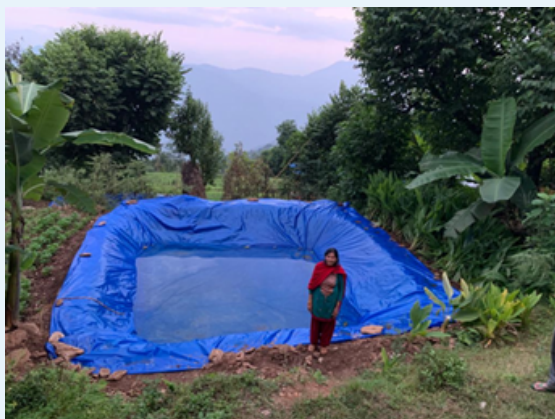
Construction of rainwater harvesting system at Siddhicharan-I, Taluwa
