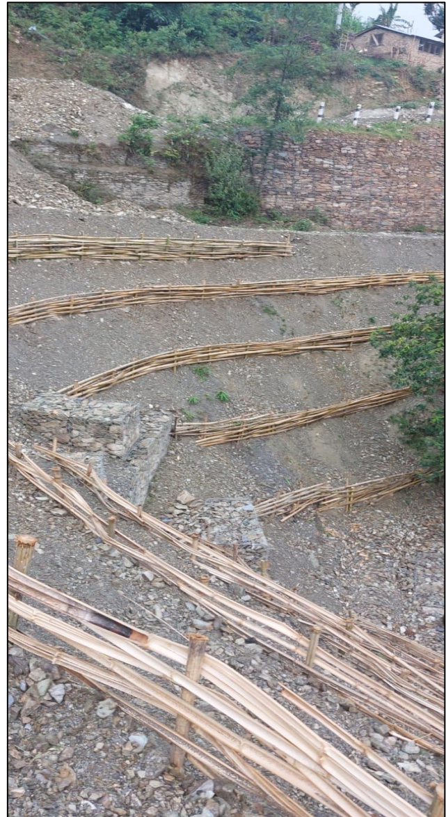
Figure 3: Downstream intervention to control soil erosion by runoff and slope stabilization
