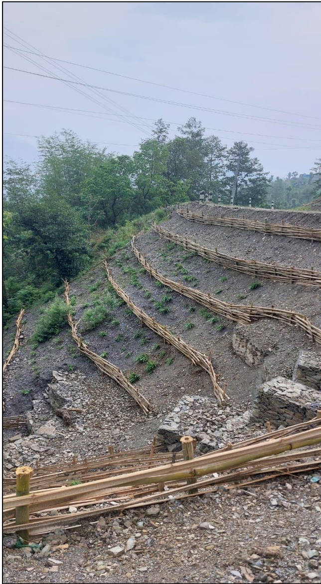
Figure 2: Downstream intervention to control soil erosion by runoff and slope stabilization
