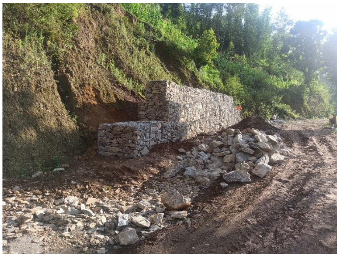
Noonthala - Jaubari road slope stabilization
