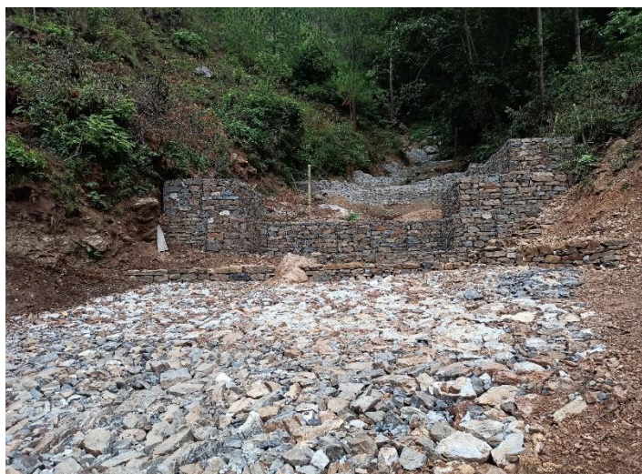
Gully Treatment work at Halesi-5, Durksem
