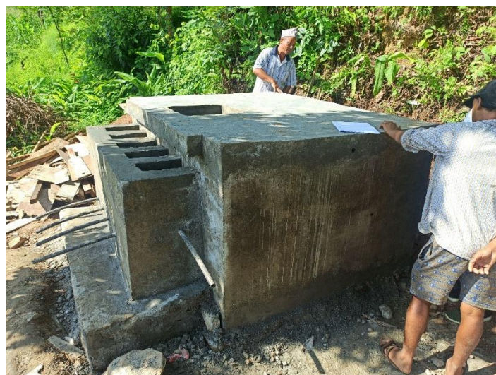
Phuli Khola water source protection work
