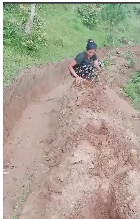
Recharge kulo Contour Trench
